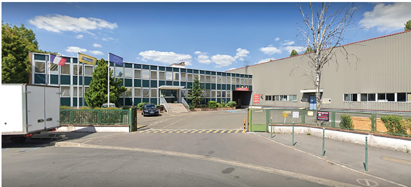
The Olaer building (now Parker) in Colombes, a suburb of Paris where I learnt “on the Gemba”
